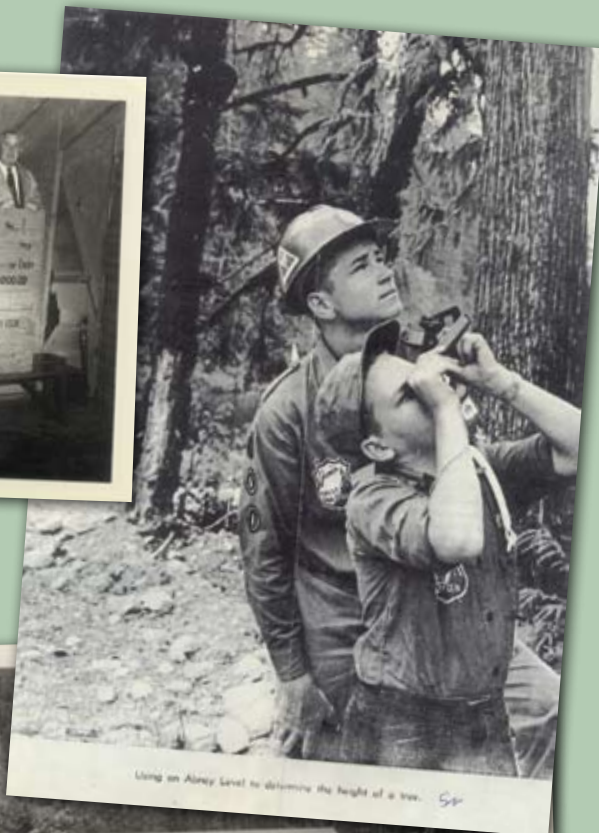
Determining the height of a tree using an Abney Level
